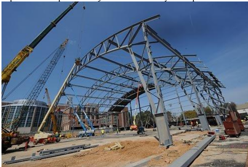
Figure 10: Structural steel erection
